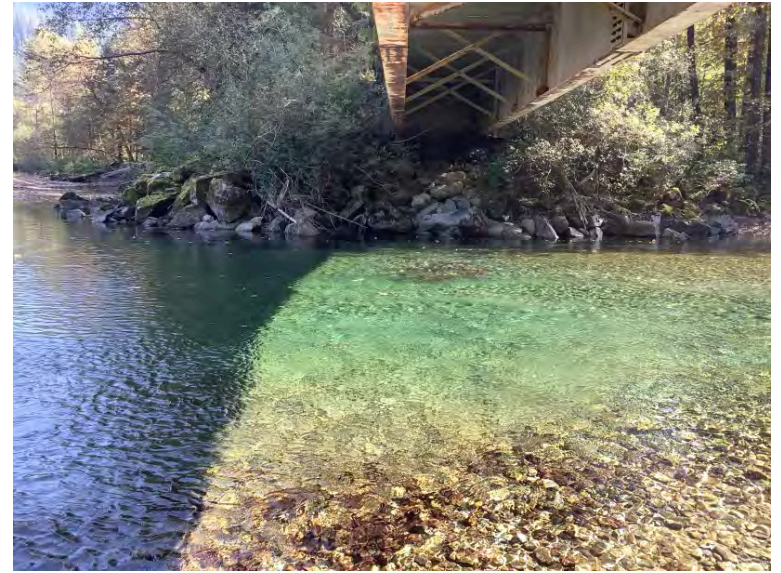
Left Bank Abutment when facing downstream
