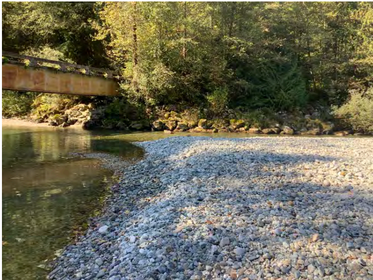
Left Bank Abutment when facing downstream
