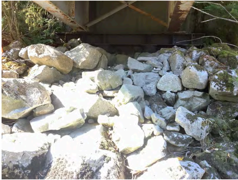
Right Bank Abutment when facing downstream
